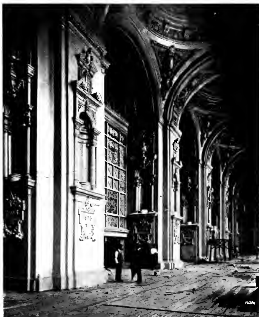
FIG. 2.—INTERIOR OF MAIN ENTRANCE, PALACE OF MACHINERY.
